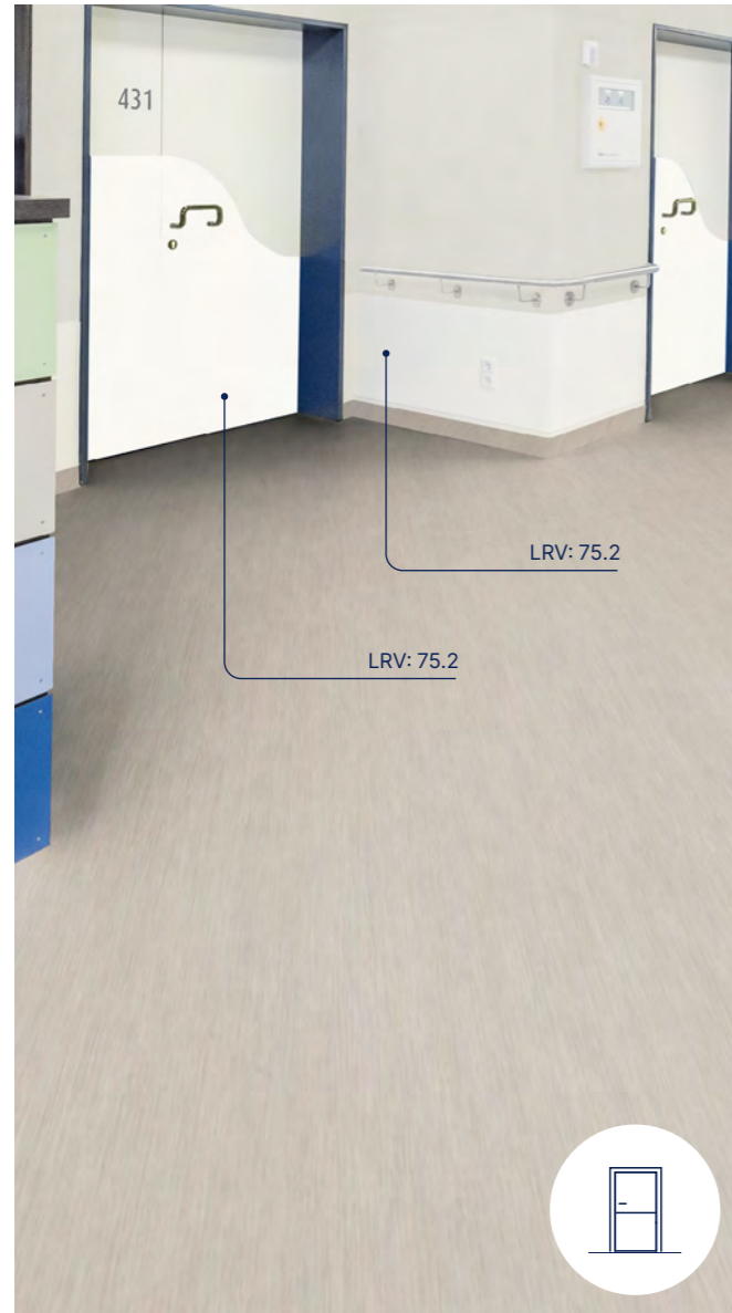
LRV differential of Wall/Door <10 points = Staff Door
