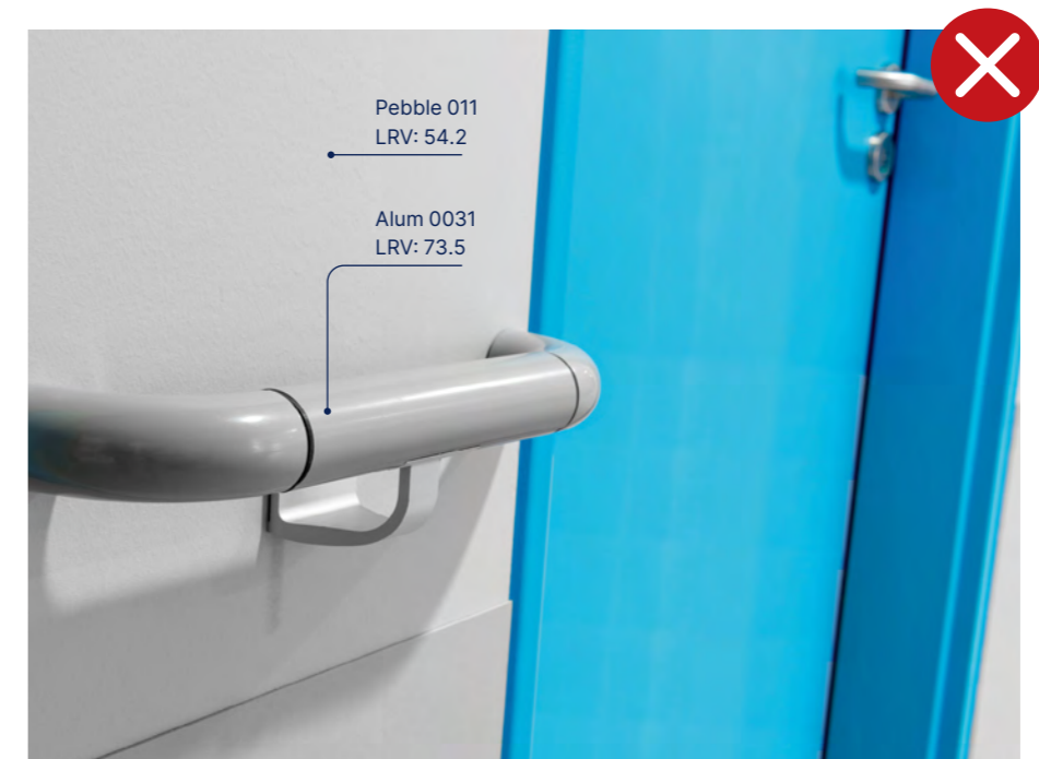
LRV differential of Wall/Handrail <30 Points
