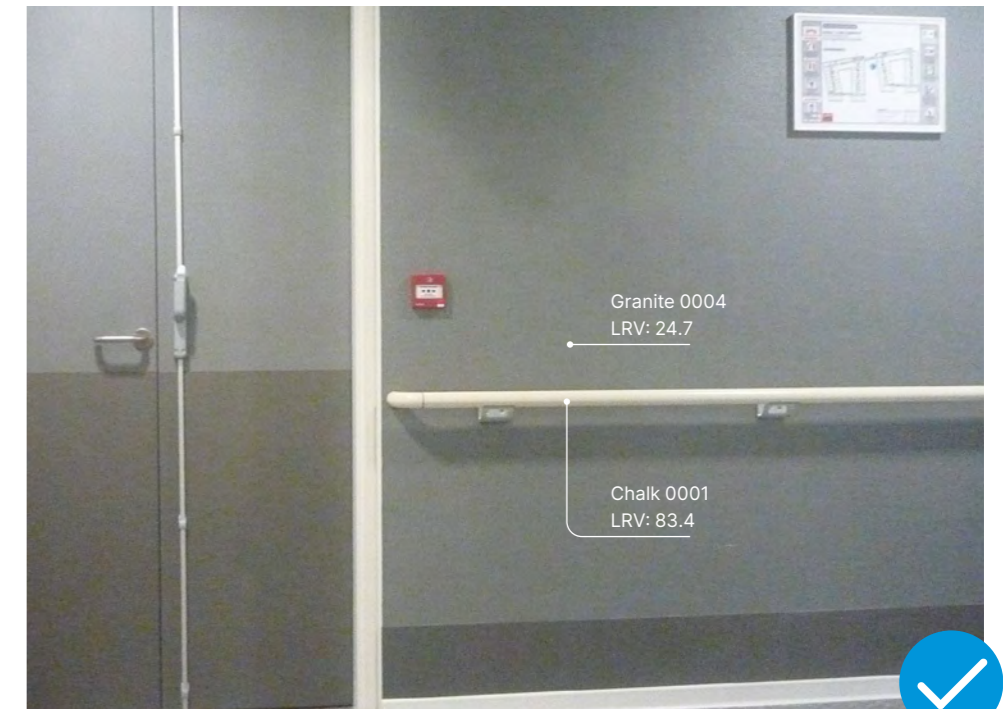
LRV differential of Wall/Handrail >30 Points
