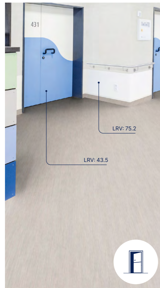
LRV differential of Wall/Door >30 Points = Public Door
